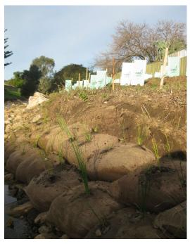
Two swales have been constructed across the slope to slow the rainwater runoff and retain soil moisture. A variety of trees, shrubs and ground covers have been planted to stabilise the soil and protect it from erosion.
