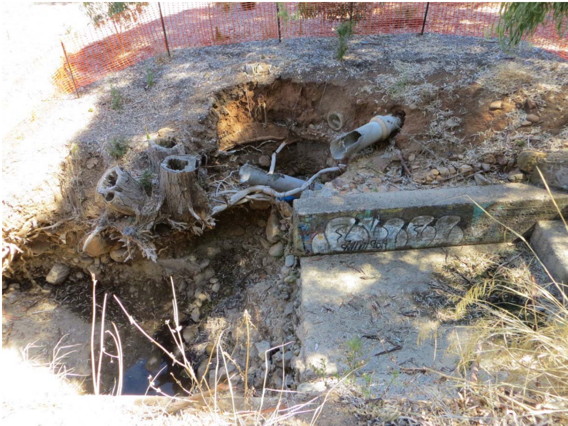
Figure 2 Erosion downstream of the Norton Summit Road bridge
