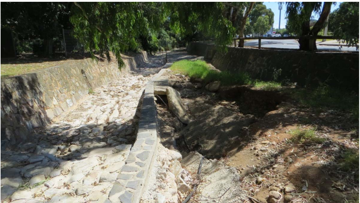
Figure 15 Erosion on the outside of the channel adjacent to Richardson Avenue
