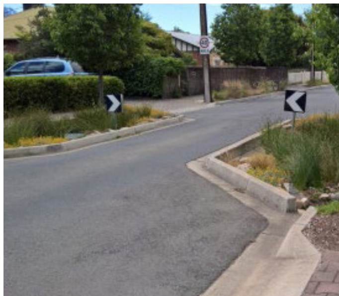
Example of slow point incorporating Water Sensitive Urban Design
