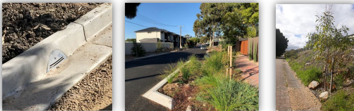
Plate 2. Examples of WSUD elements: street tree inlet, biofiltration and porous stoneset
