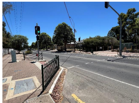
Pedestrian actuated crossing adjacent Thorndon Park Primary School in Stradbroke Road, Athelstone with a 60 km/h speed limit
