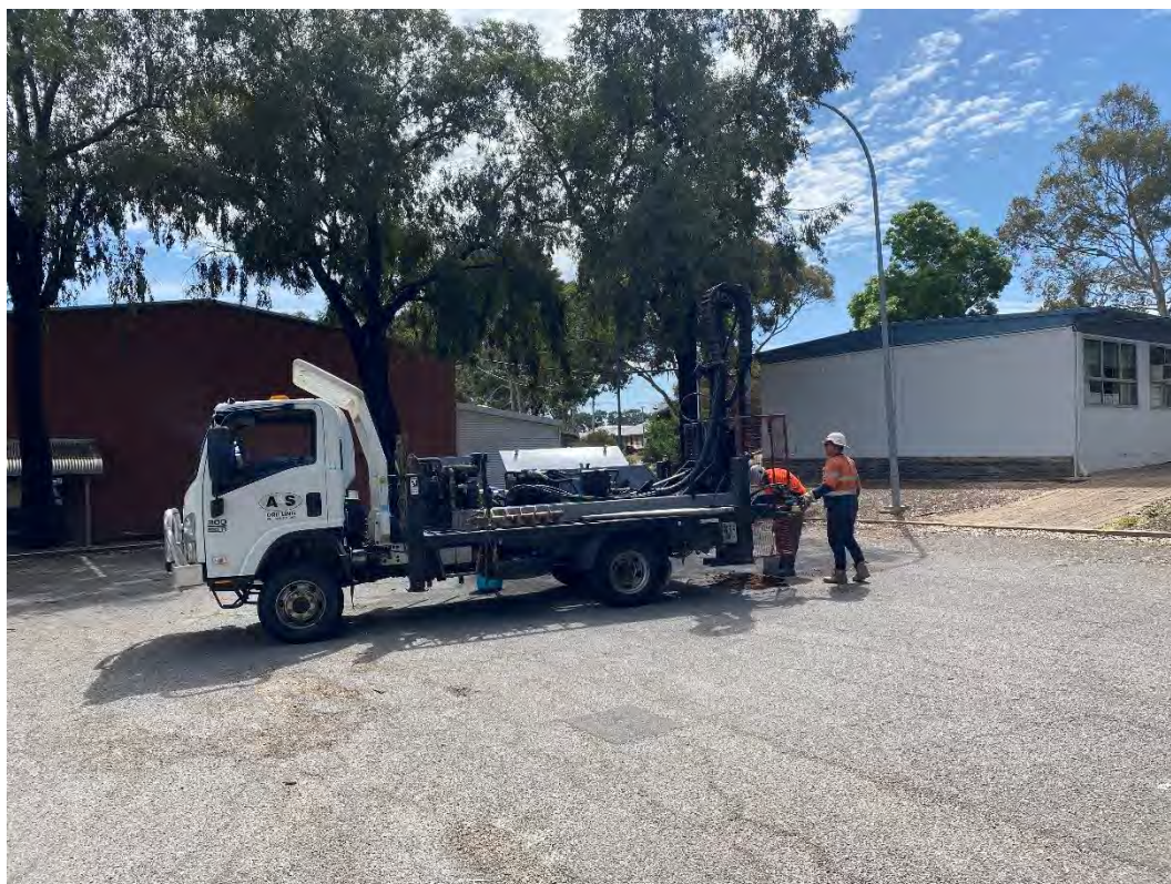
Figure 3: Site photograph at BH05, Rostrevor High School (06-10-21)
