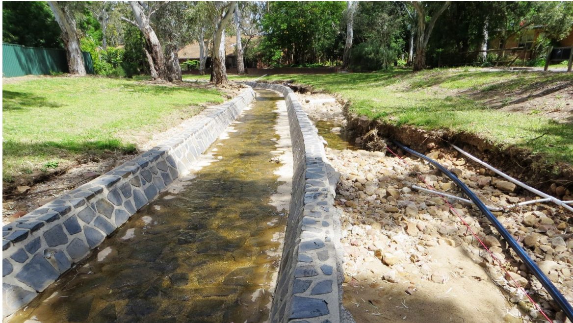
Figure 7 Erosion either side of the concreted channel has undermined the concrete and exposed pipework, November 2016
