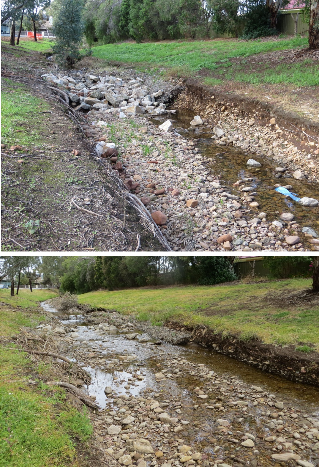
Figure 13 Example of instream rock structure in subsection 8 that was beginning to fail at the downstream end in May 2016 (top), however this was covered in rocks during the floods, reducing the erosion at this site (bottom).
