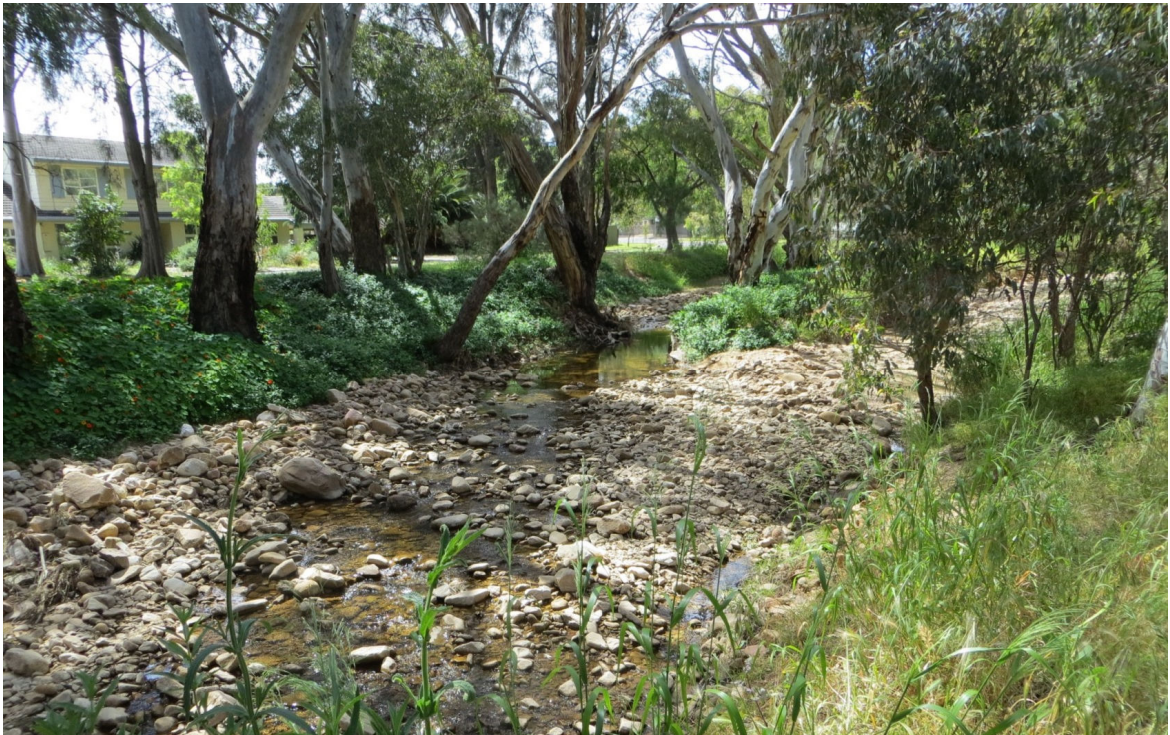
Figure 5 Showing the channel bed scoured clear of sediment and vegetation in November 2016 but without bed deepening
