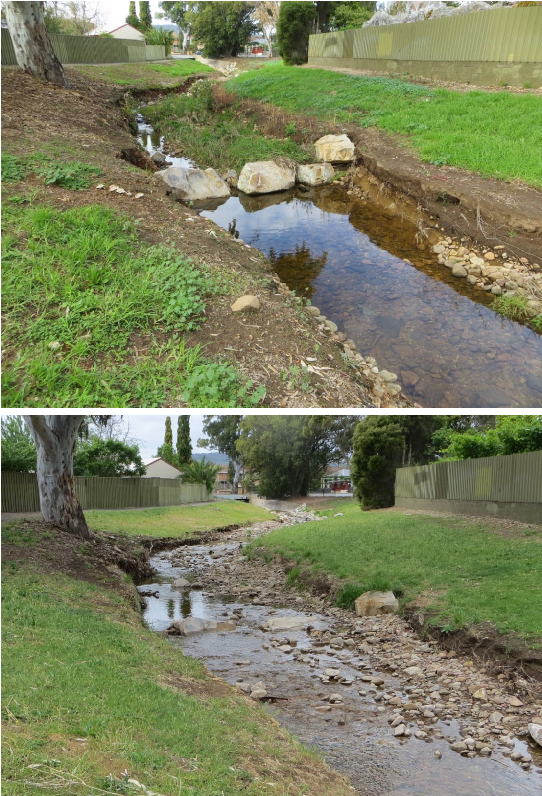
Figure 16 Showing an area in lower subsection 7 impacted by bed deepening and erosion around the rock weir in May 2016 (top) where bed materials from upstream were deposited during the floods (bottom)
