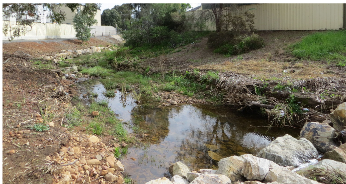
Figure 12 Downstream end of subsection 7 in May 2016, revegetation area on right bank in background without spraying, rocks placed in creek to raise bed level in foreground and on left bank downstream to prevent channel widening
