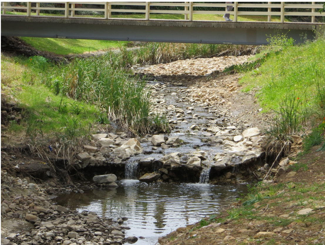
Figure 11 Upstream end of subsection 6 following the 2016 floods; the top layer of sediment and rock has been removed upstream of a concrete weir, along with Bulrushes and Blackberries, but the weir has prevented bed deepening below this level.
