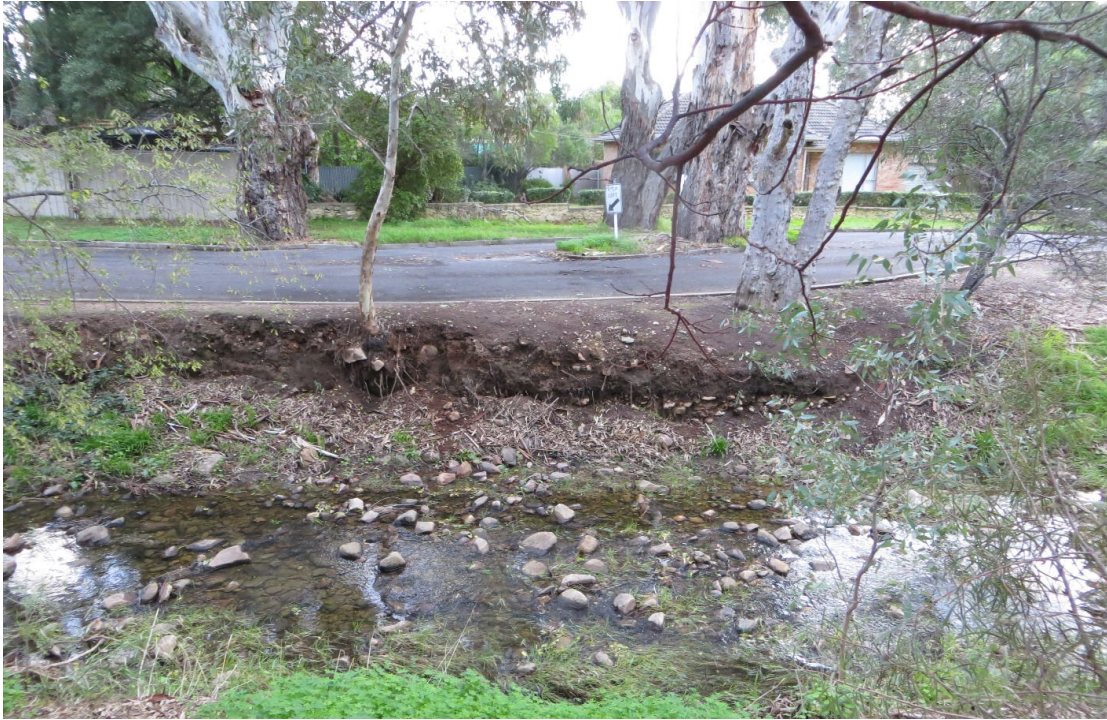
Figure 17 Bank erosion in subsection 2; because of the narrow width, controlling this erosion is important for protecting the road
