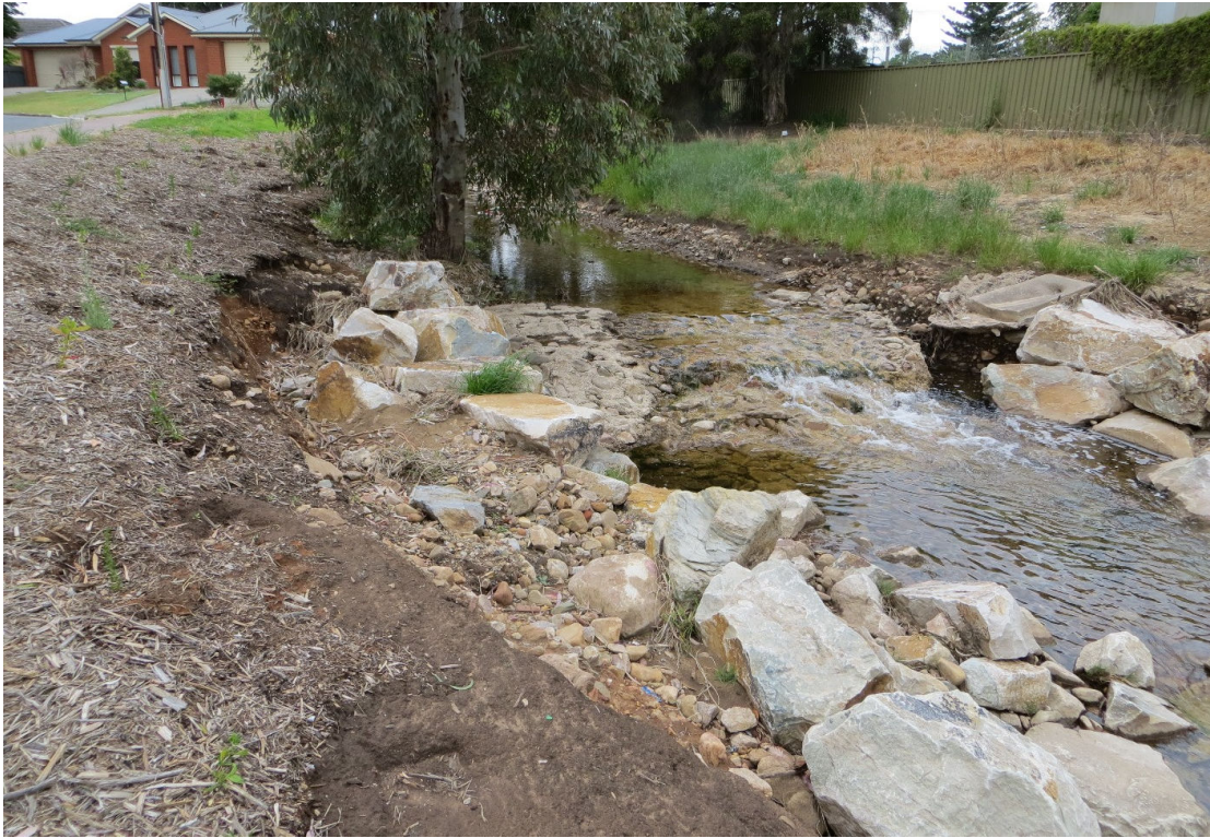
Figure 10 National Tree Day 2016 planting site to the left; the instream concrete weir has prevented bed deepening but minor scouring around the structure has occurred
