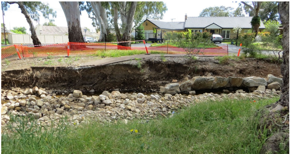
Figure 2 Erosion of the banks leading to loss of the footpath. Note large rocks that have been placed here prior to the 2016 floods indicate the previous channel alignment.
