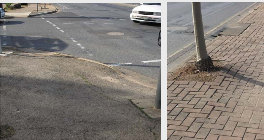
6. Non-compliant pram ramps and uneven footpath surfaces
