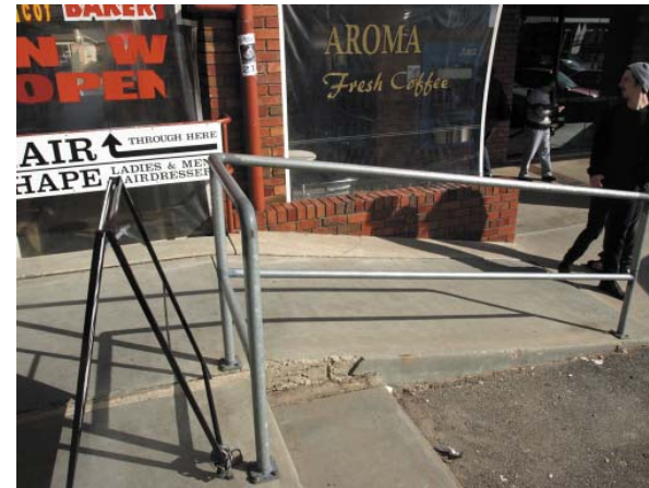
1. Non-compliant ramp + hand rails
