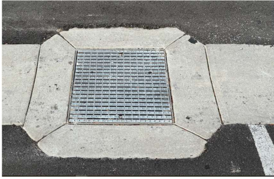
Grated Inlet Pit
