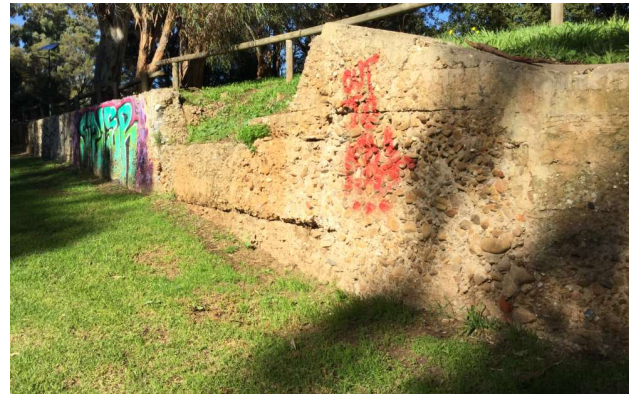
River Drive – Asset ID 119714
