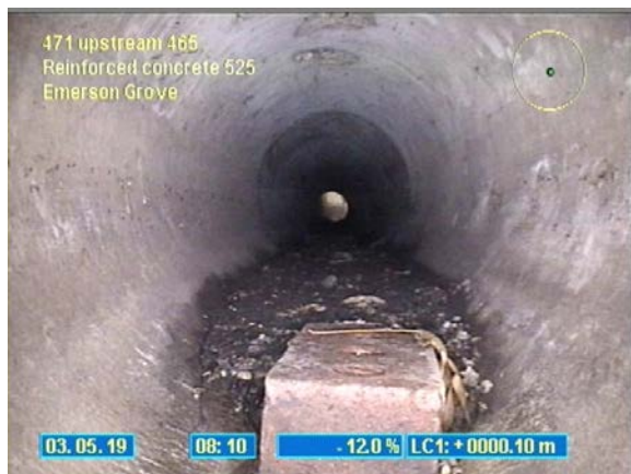
Deposit of the debris obstructing the flow
