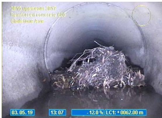
Deposit of the debris obstructing the flow
