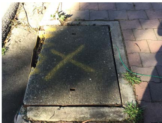
Expired pit cover that require replacement
