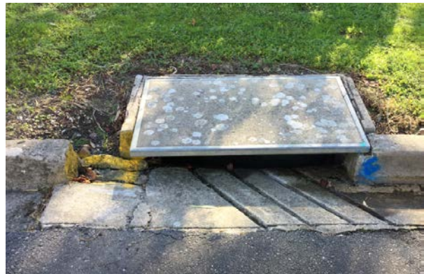
Pit cover surrounding (kerb) damage
