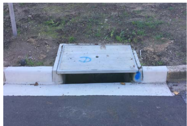
example of a recently repaired pit (cover and its surroundings)
