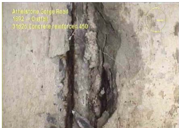
Spalling of concrete at a pipe joint
