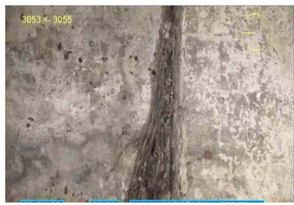
Pipe joint displacement due to root intrusion
