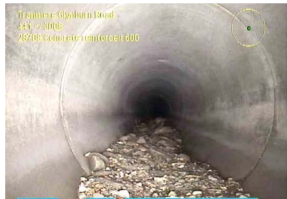
Deposit of the debris obstructing the flow
