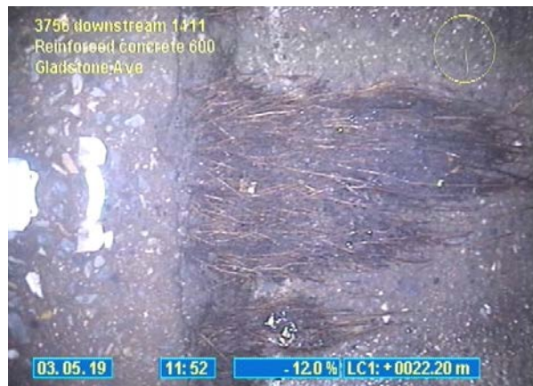
Pipe joint displacement due to root intrusion
