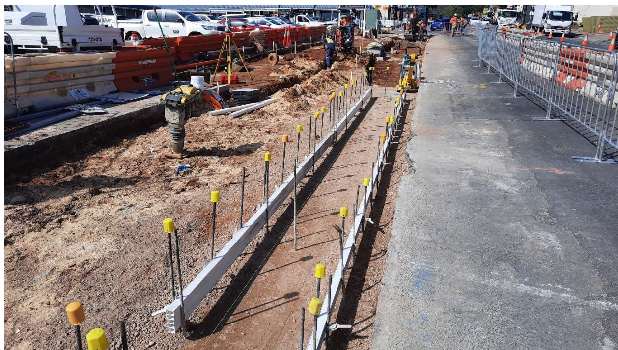
Figure 5: Kerb and Footpath Preparation Works Stage 3
