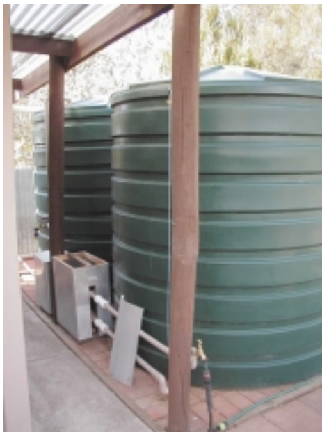
Photo: rainwater tanks can be used to water the garden - they are also great to plumb into the bathroom and laundry to save water inside your home.
