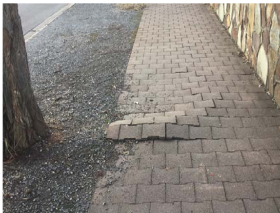
Tree roots causing paver lifts
