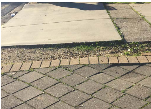
Missing sections of footpath
