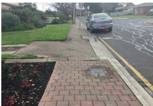
Depression caused water ponding
