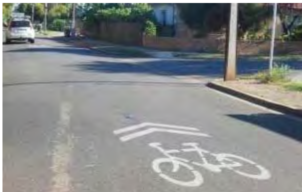
Figure 5.1: Example of Sharrow Treatment
